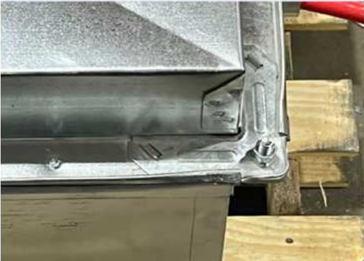
FIGURE J – Corner bolts wrench tight 25 ft.lb
