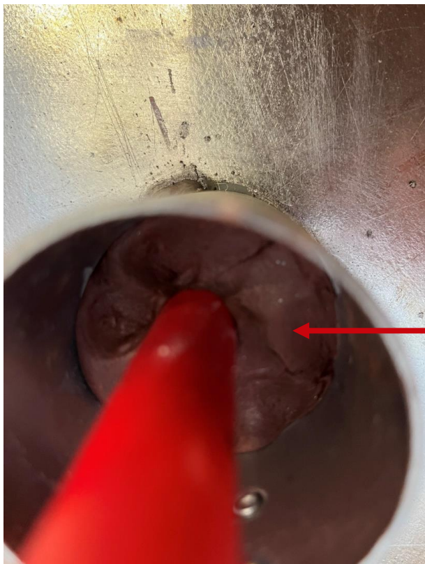
FIGURE H – Sleeve Firestop
