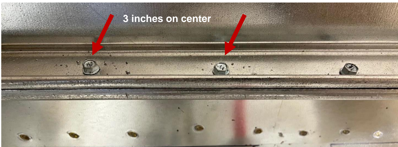
FIGURE K – #10 sheet metal screws 3" o.c.
