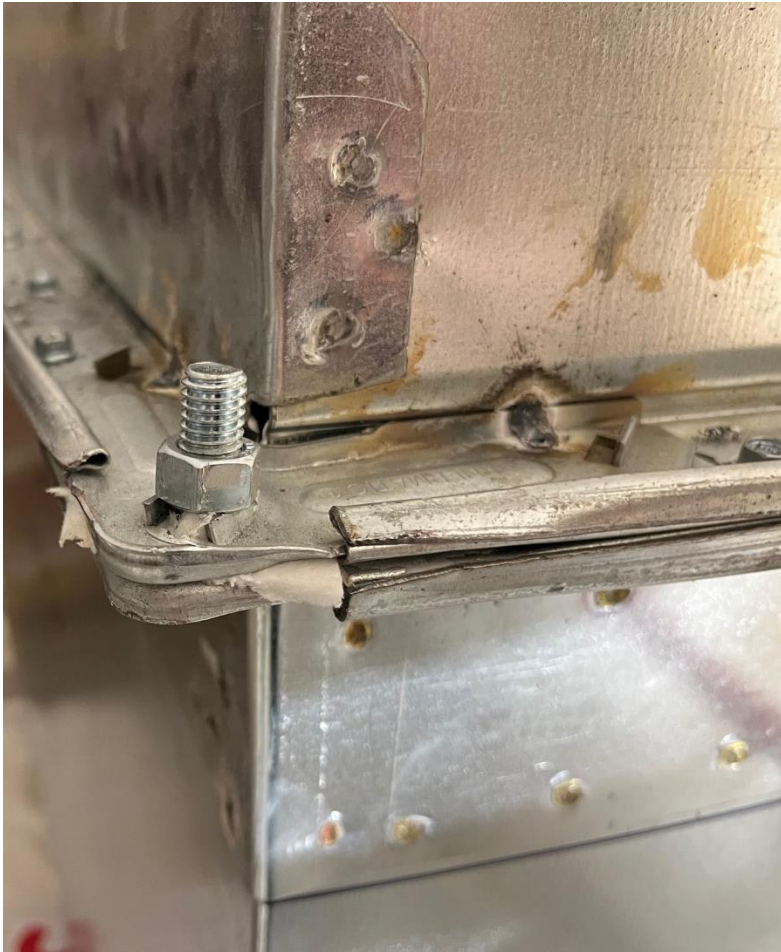
FIGURE J – Corner bolts wrench tight 25lbs
