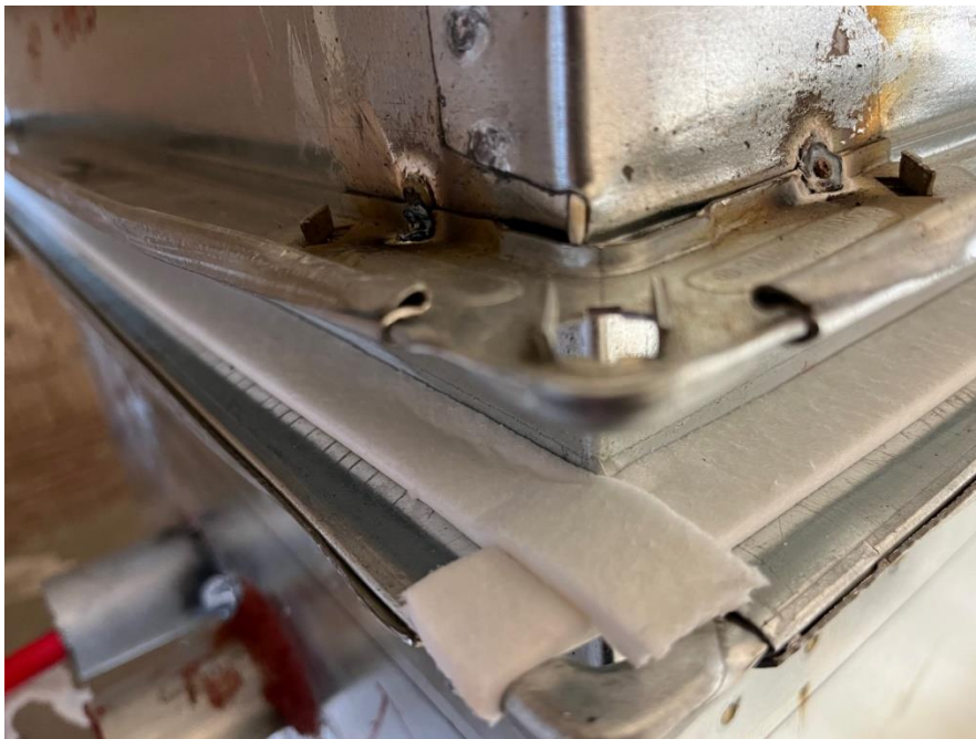
FIGURE I – Factory Installed Gasket
