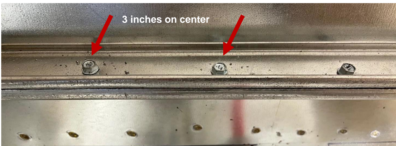
FIGURE K – #10 sheet metal screws 3" o.c.
