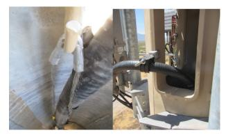
Once the hybrid cable is hoisted to the appropriate height, anchor it to the support structure, starting at the top.
