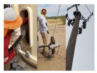
Due to the DC wire, hybrid cable is heavier than traditional cable; use a strong pulley at both the top and bottom of the tower to guide the hoist line. A minimum of persons is needed to properly hoist the cable assembly.
